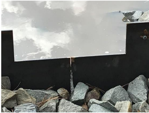
Figure 2. Examples of discharge structure configurations. A. 2-stage weir plate, B. Riser pipe with orifices C. Flash board riser and D. Riser constructed of masonry blocks with gaps between blocks.
