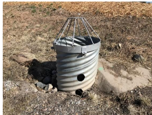
Figure 2. Examples of discharge structure configurations. A. 2-stage weir plate, B. Riser pipe with orifices C. Flash board riser and D. Riser constructed of masonry blocks with gaps between blocks.
